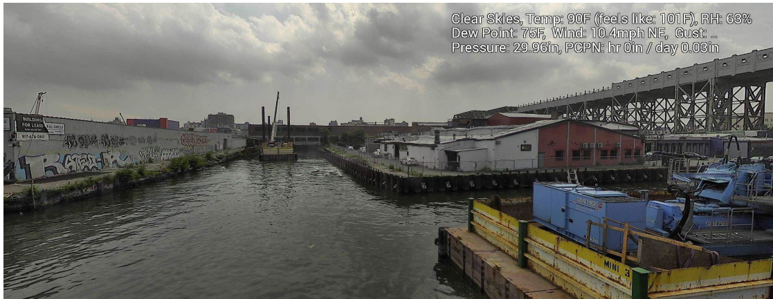
Figure 8 – July 31, 2025. General Conditions in Canal north of 9 th Street Bridge near TB7 during in-waterway construction activities.
