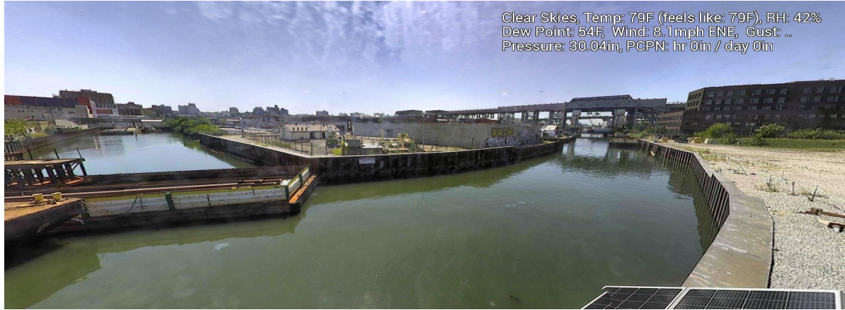
Figure 10 – August 22, 2025. General Conditions in Canal north of 9 th Street Bridge near TB6 during in-waterway construction activities.
