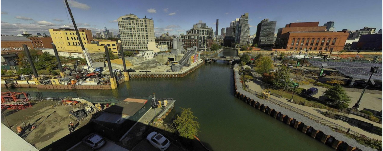
Figure 10 – October 23, 2025. Conditions observed south of 3rd Street Bridge during midday.
