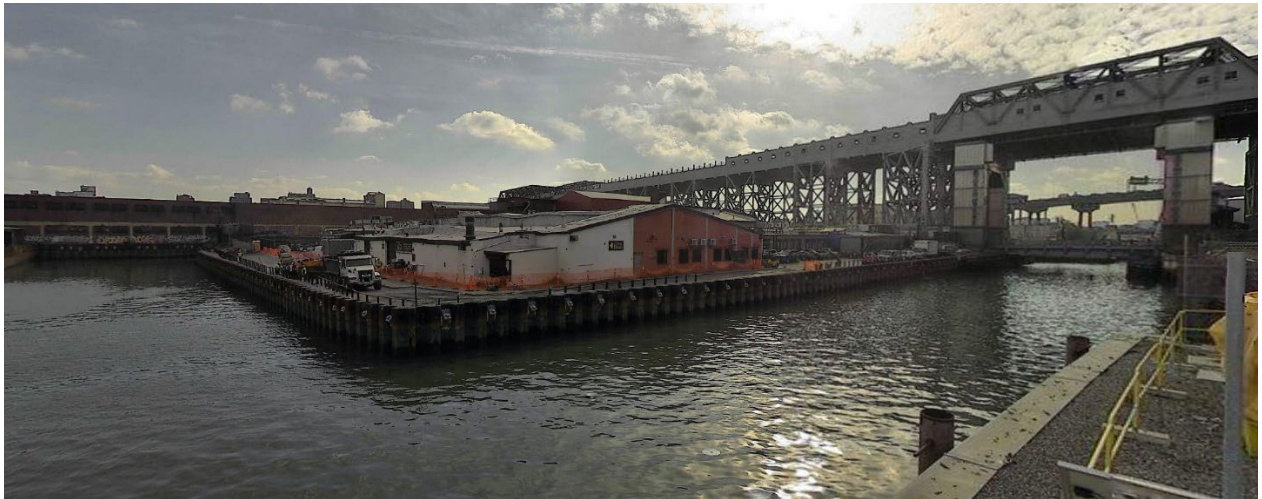
Figure 9 – December 4, 2025. Midday conditions near Turning Basin 7 and the main canal, north of 9 th Street Bridge.
