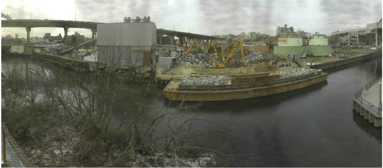
Figure 9 – January 2, 2026. Midday conditions south of the Ninth Street Bridge.
