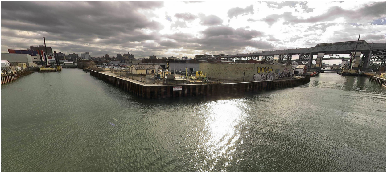
Figure 9 – January 7, 2026. Midday conditions near Turning Basin 6 and the main canal, north of 9 th Street Bridge.
