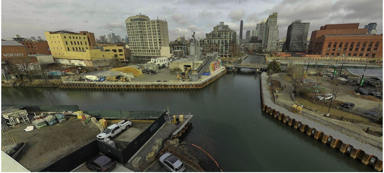
Figure 12 – January 9, 2026. Midday conditions near 3 rd Street Bridge and Turning Basin 4.
