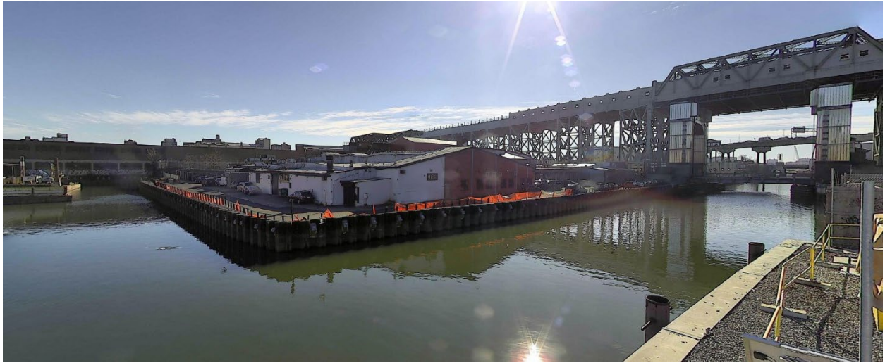
Figure 8 – January 12, 2026. Midday conditions near Turning Basin 7 and the main canal.
