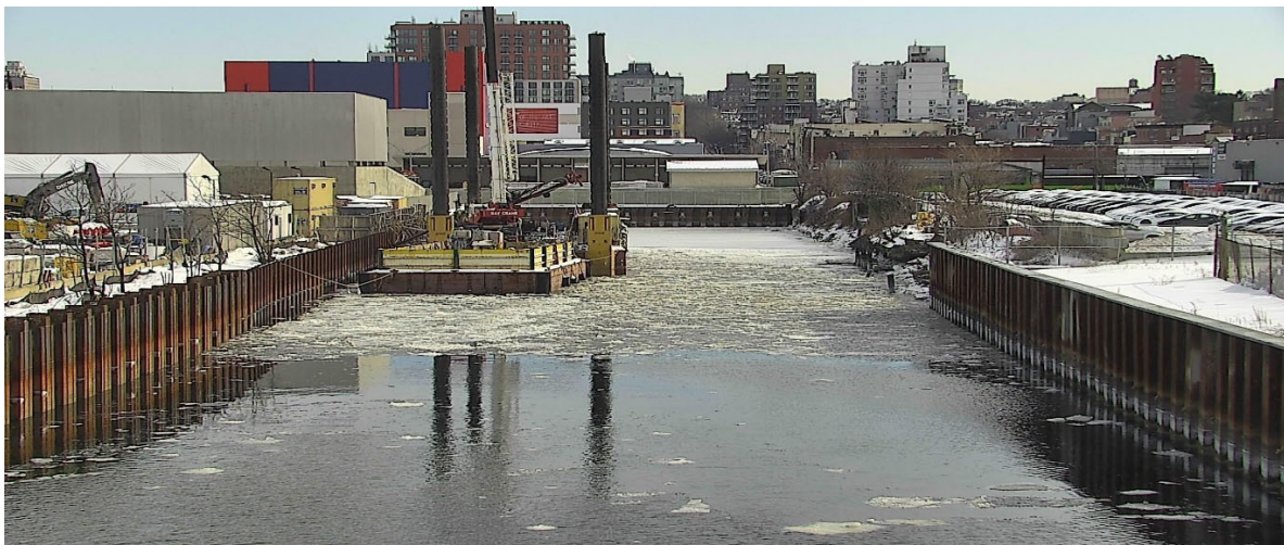
Figure 8 – January 27, 2026. Midday conditions near Turning Basin 6 and the main canal.
