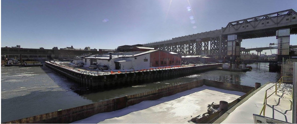
Figure 7 – January 30, 2026. Midday conditions near Turning Basin 7 and the main canal.
