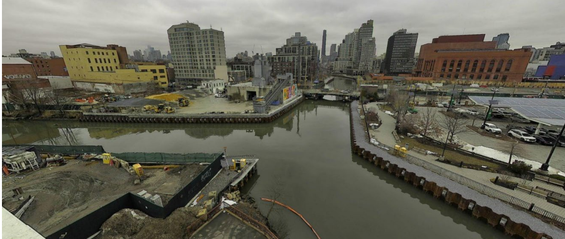
Figure 10 – March 6, 2026. Midday conditions near Turning Basin 4 and the main canal.
