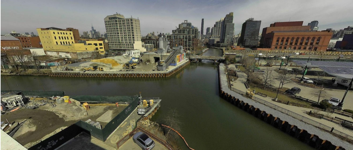
Figure 10 – March 20, 2026. Midday conditions near Turning Basin 4 and the main canal.
