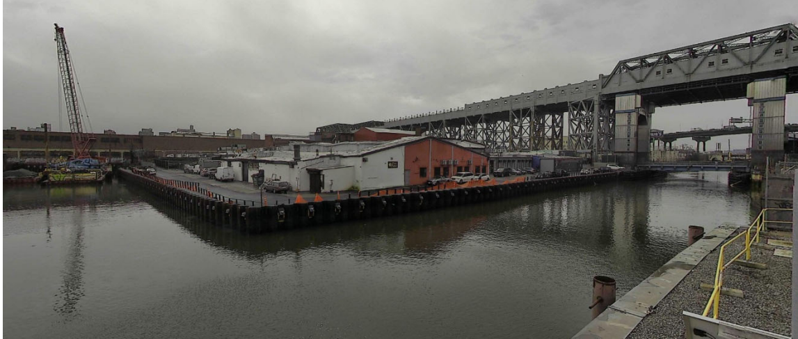
Figure 8 – March 16, 2026. Midday conditions near Turning Basin 7 and the main canal.
