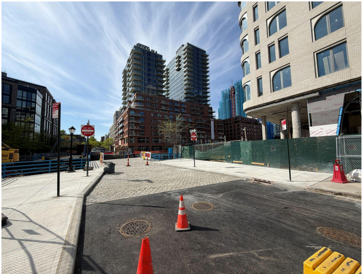
Restoration of the roadway.
