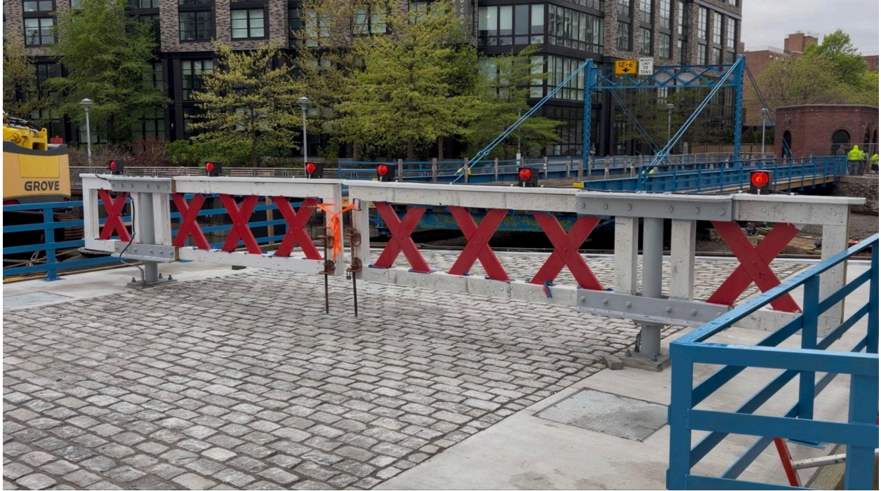
Installed traffic gates.
