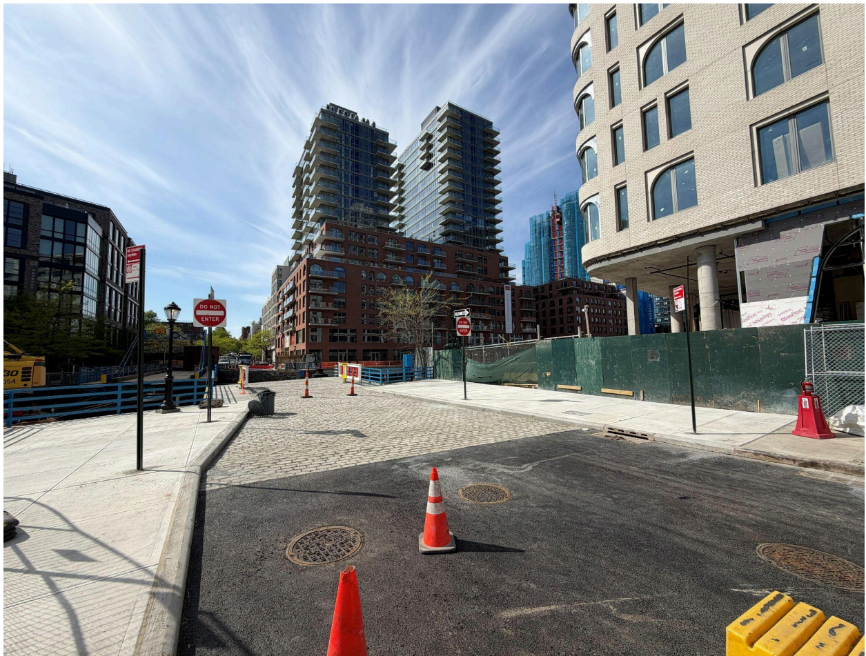
Restoration of the roadway.
