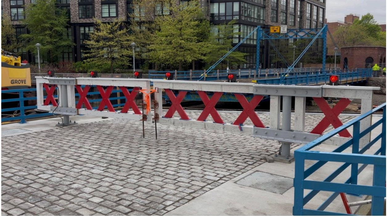
Installed traffic gates.
