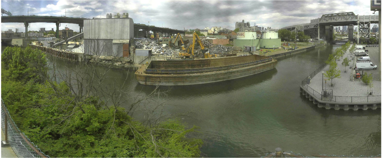
Figure 10 – May 8, 2026. Midday conditions between Hamilton Street Bridge and 9 th Street Bridge
