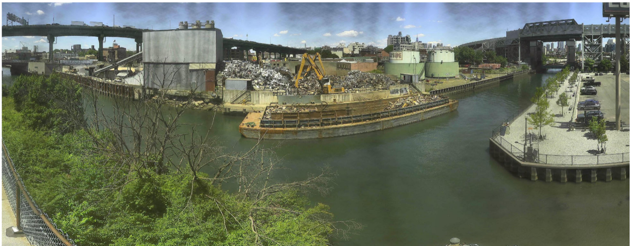
Figure 9 – June 24, 2026. Midday conditions between Hamilton Street Bridge and 9 th Street Bridge.
