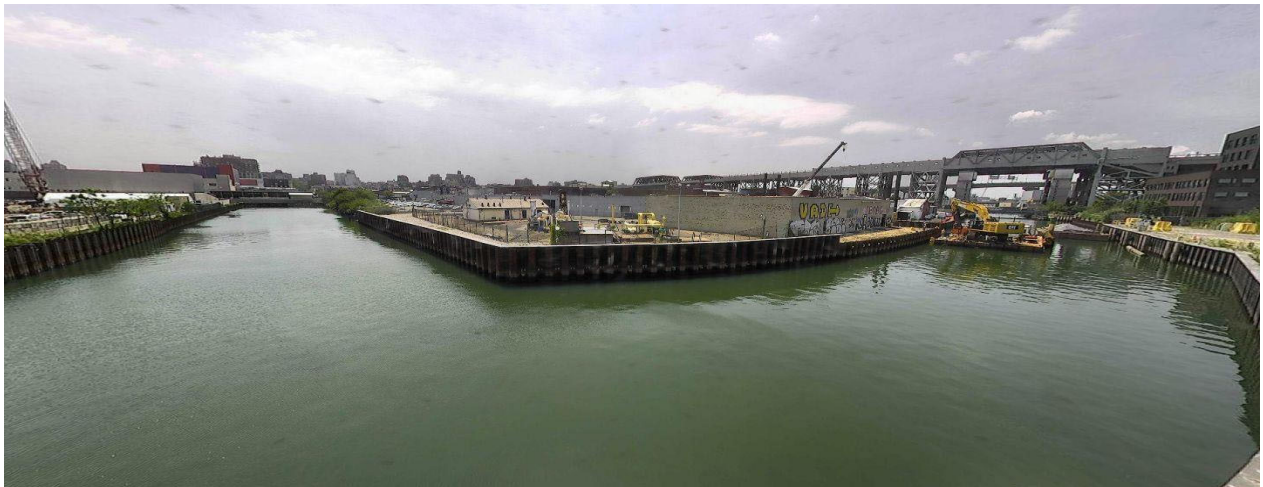
Figure 8 – June 30, 2026. Midday conditions between North of 9 th Street bridge near turning basin 6.
