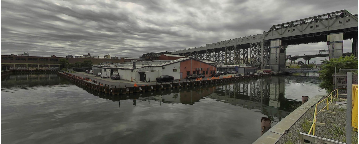
Figure 10 – August 5, 2026. Midday conditions North of 9 th Street Bridge near Turning Basin 7.
