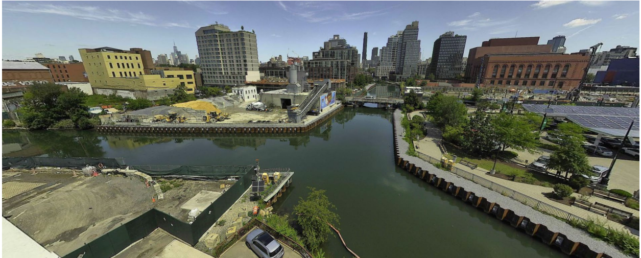
Figure 8 – August 4, 2026. Midday conditions south of 3 rd Street Bridge.
