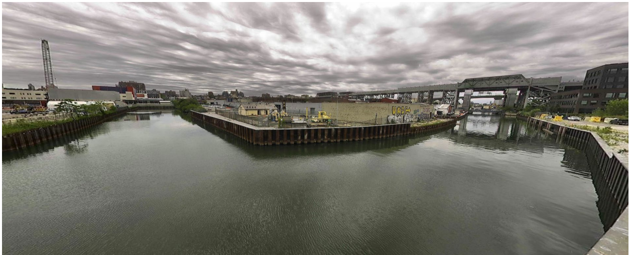
Figure 9 – August 5, 2026. Midday conditions North of 9 th Street Bridge near Turning Basin 6.
