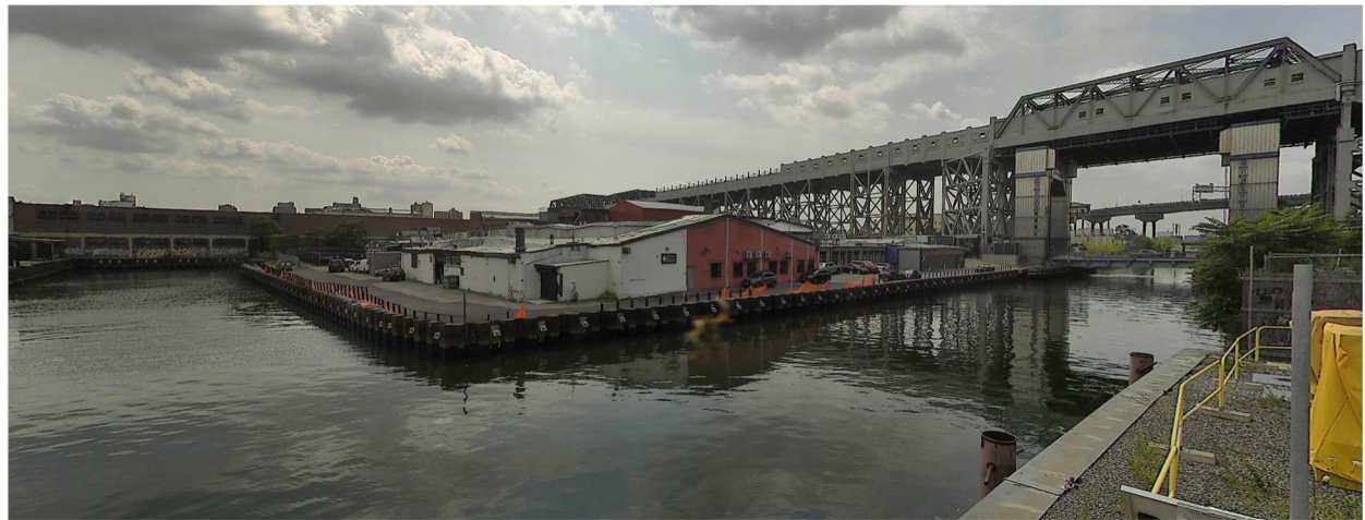
Figure 9 – August 13, 2026. Midday conditions North of 9 th Street Bridge near Turning Basin 7.
