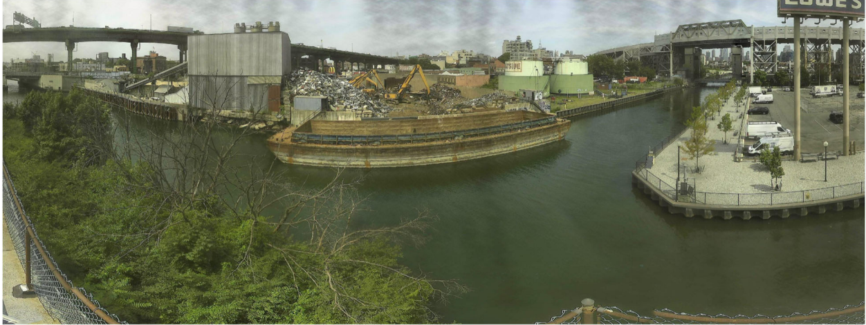
Figure 10 – August 14, 2026. Midday conditions between 9 th Street Bridge and Hamilton Street Bridge.
