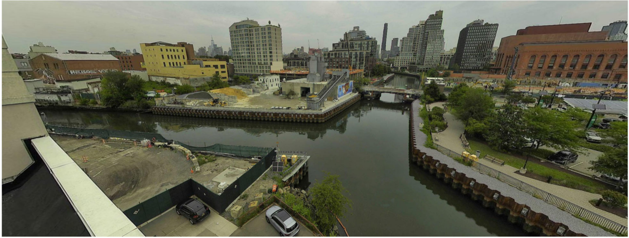
Figure 8 – August 10, 2026. Midday conditions south of 3 rd Street Bridge.
