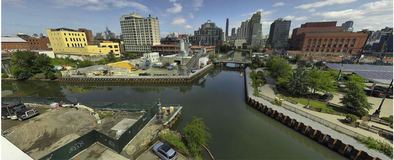
Figure 10 – August 21, 2026. Midday conditions south of 3 rd Street Bridge.
