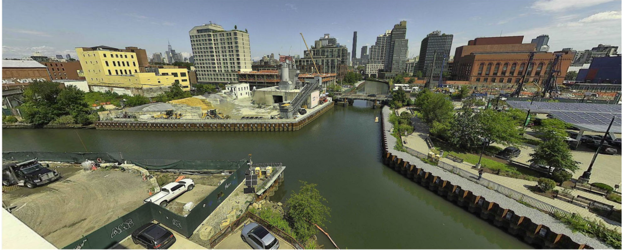
Figure 8 – August 24, 2026. Midday conditions south of 3 rd Street Bridge.
