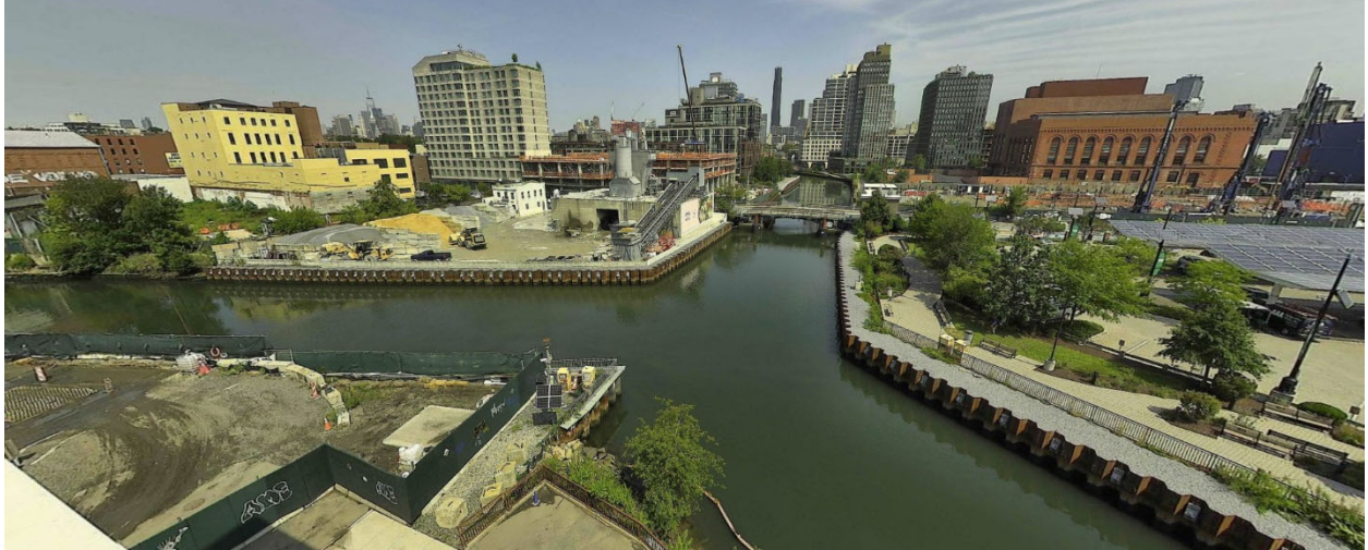
Figure 10 – August 28, 2026. Midday conditions south of 3 rd Street Bridge.
